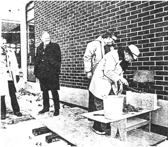
Board Chairman Arthur Stoll lays the cornerstone.
